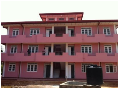
Re-Construction of Consultant Quarters, DGH Mannar.
