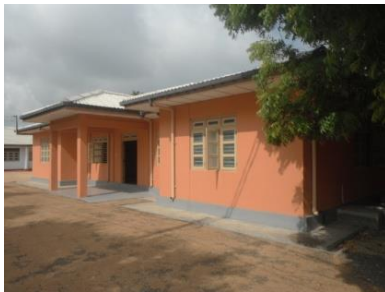
Refurbishment of RMO/AMC Office at Pannai - Jaffna
