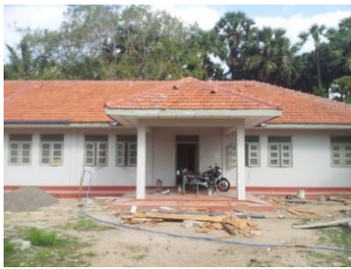
Re-Construction of MOH Office,Velanai-Jaffna
