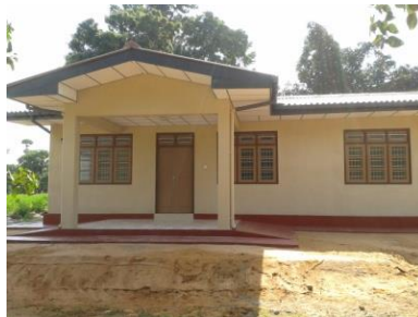
Construction of MO Quarters, Palai- Kilinochchi
