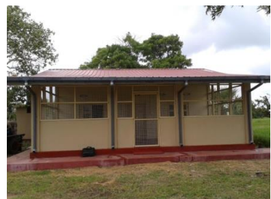
Renovation & Repairs of GHC at Thampirai-Kilinochchi
