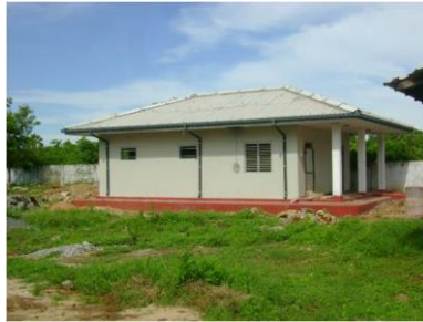
Re-Construction of Mortuary Block at DH,Atchuvvely-Jaffna
