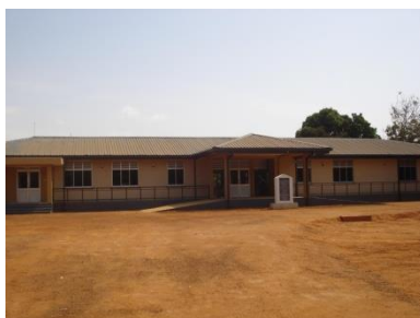
Construction of OPD Block, Mulankavil-Kilinochchi
