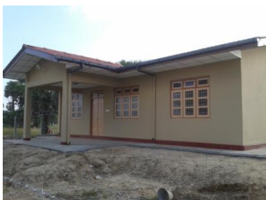
Construction of MO Quarters, Palai-Kilinochchi
