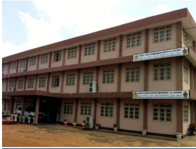
Re-construction of Regional Training Centre(Stage iv), Pannai-Jaffna
